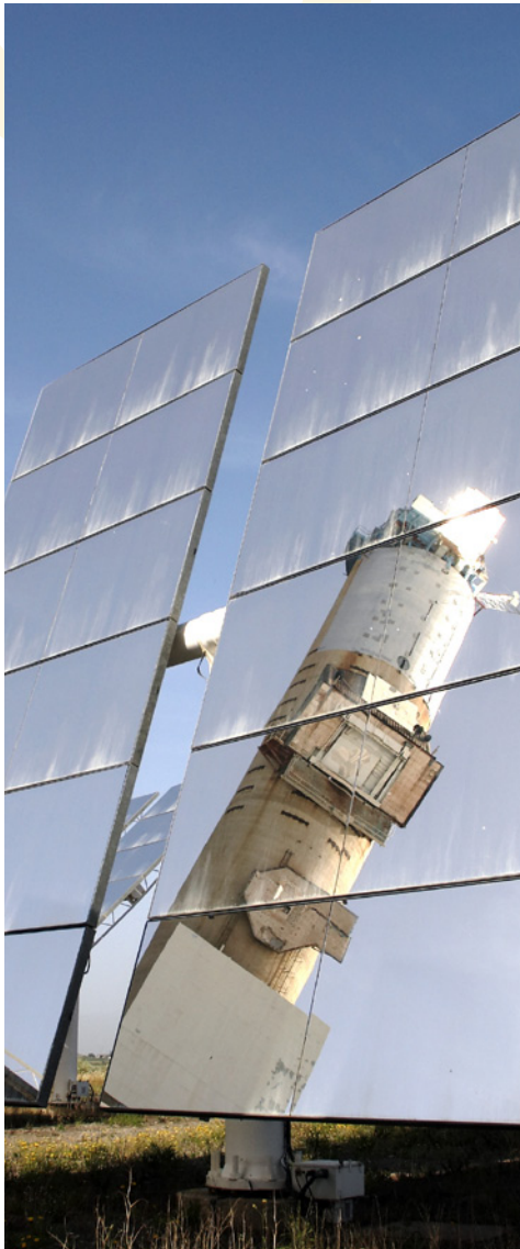
Almería Solar Platform. Singular Scientific and Technical Infrastructure (ICTS)
